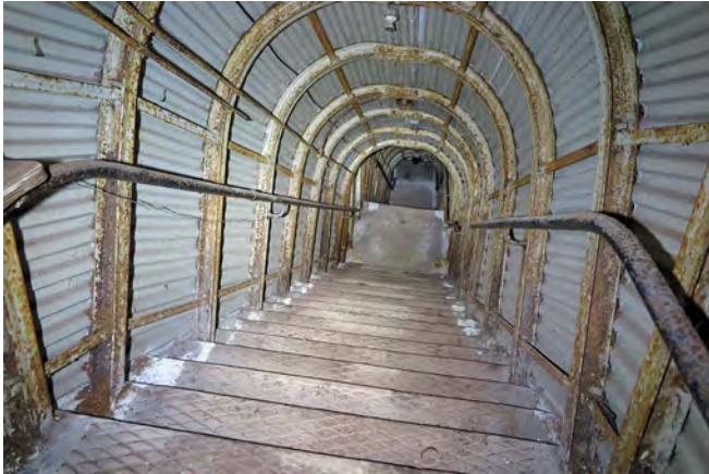
Staircase at Fort Southwick which would have formed the original entrance to the tunnel complex.
